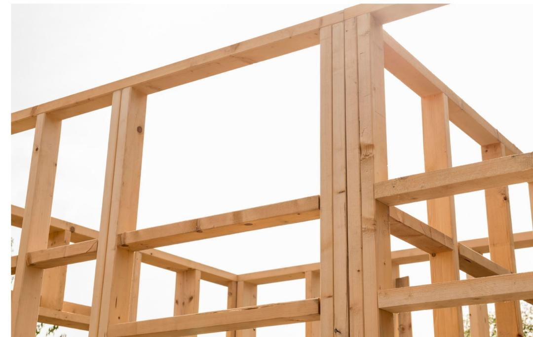
*Figure 9. Timber frames for lightweight cladding.*
