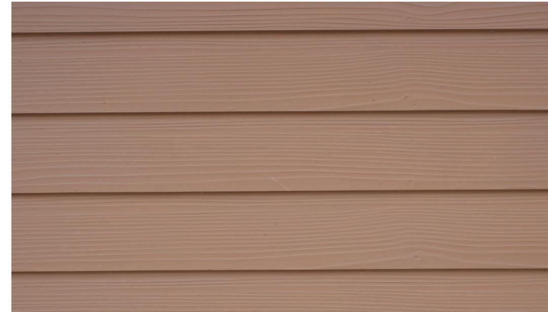
*Figure 8. Fiber cement for lightweight cladding.*
