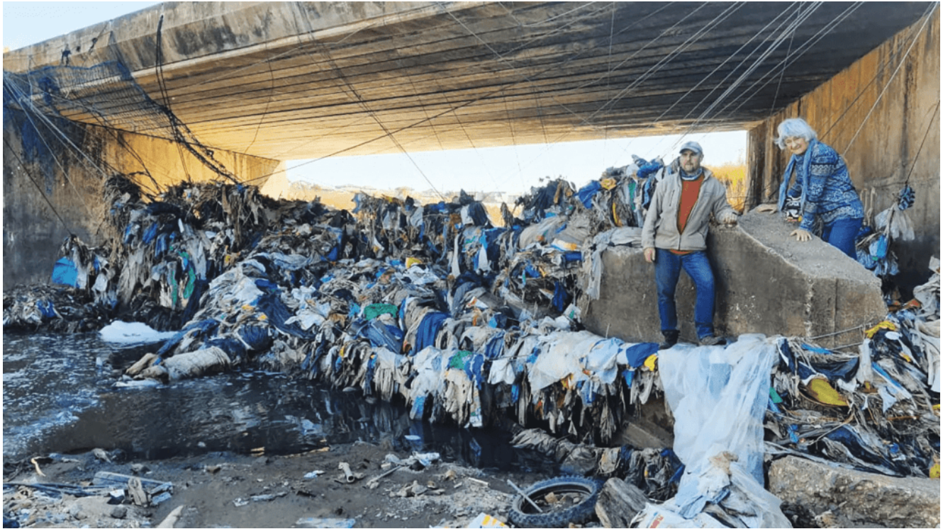
A river-trap built by the NGO Armour, to stop waste from flowing into the Hennops River (South Africa).
